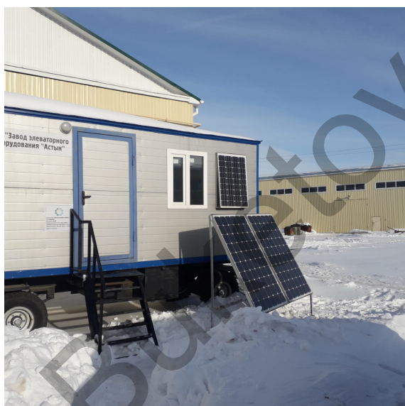
Fig.2. Solar plant: a) solar panels; b) batteries, controller, inverter
