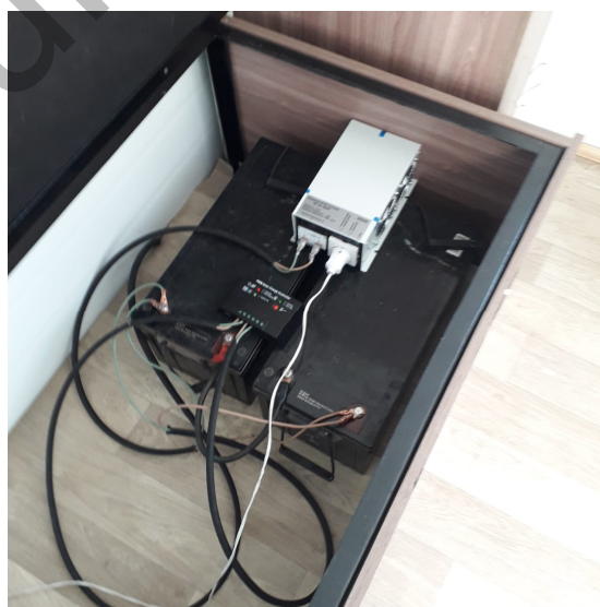
Fig.2. Solar plant: a) solar panels; b) batteries, controller, inverter
