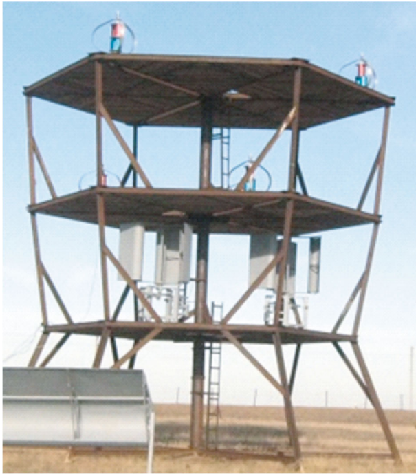
Fig. 1. Prototype of a CTWPP with a power of 3 kW.
