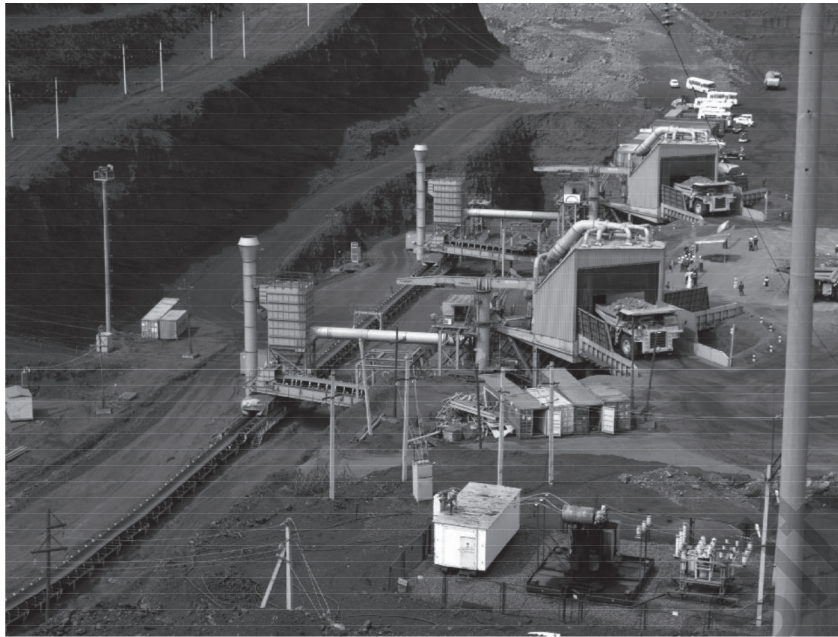
Figure 2 Cyclic-flow technology at the Vostochny open-pit mine
