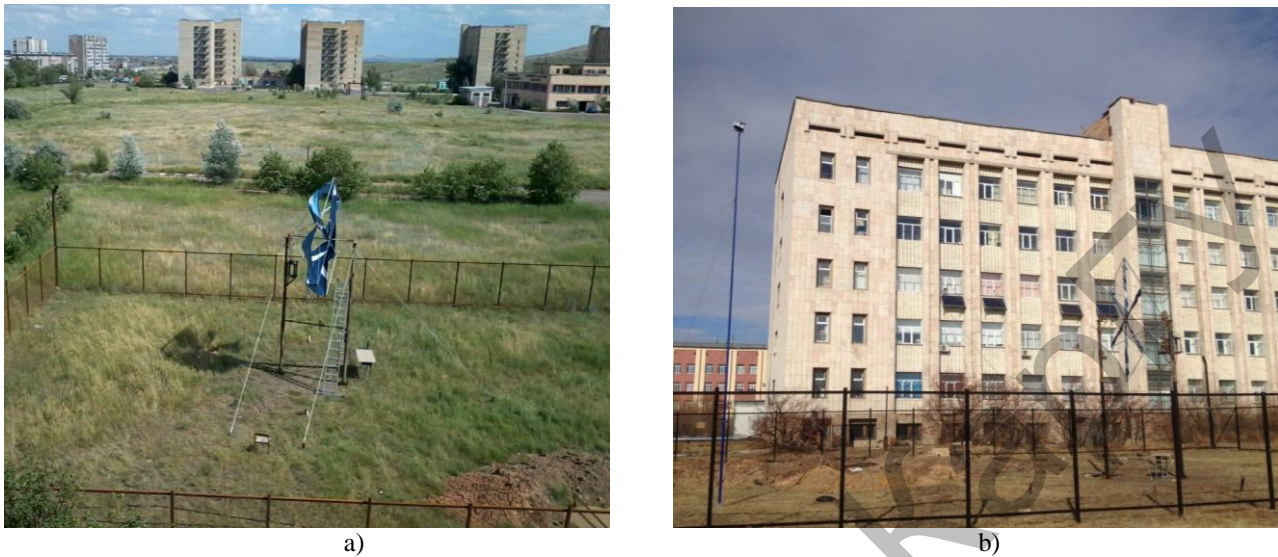
Fig.7. General view of WT-4 wind turbine: a) operational mode, b) - idle mode (sail blades are taken in)
