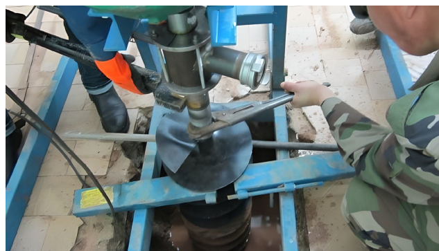
Fig. 3. Installation of suspended Equipment
