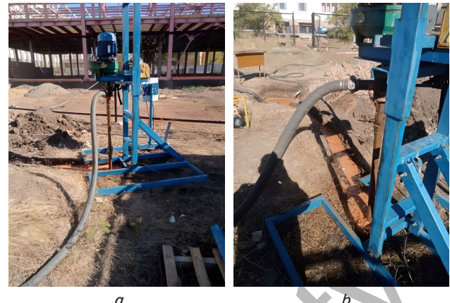
Fig. 5. Small drilling rig
